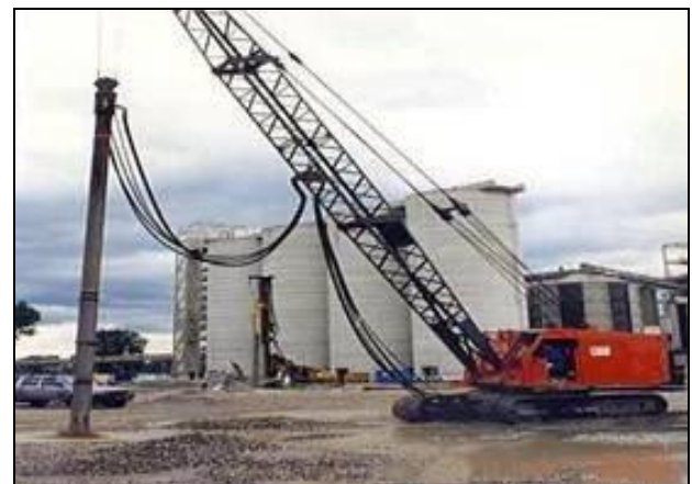
Fig 2: Vibro-Compaction Method
