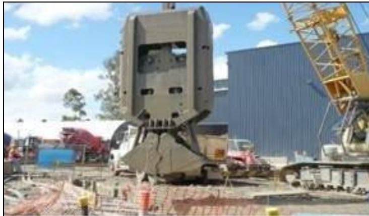
Fig 3: Vacuum Consolidation of Soil
