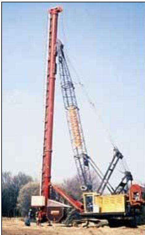
Fig 1: Vertical Drain
