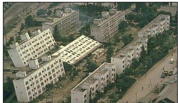
**Fig 1:** Some effects of liquefaction
